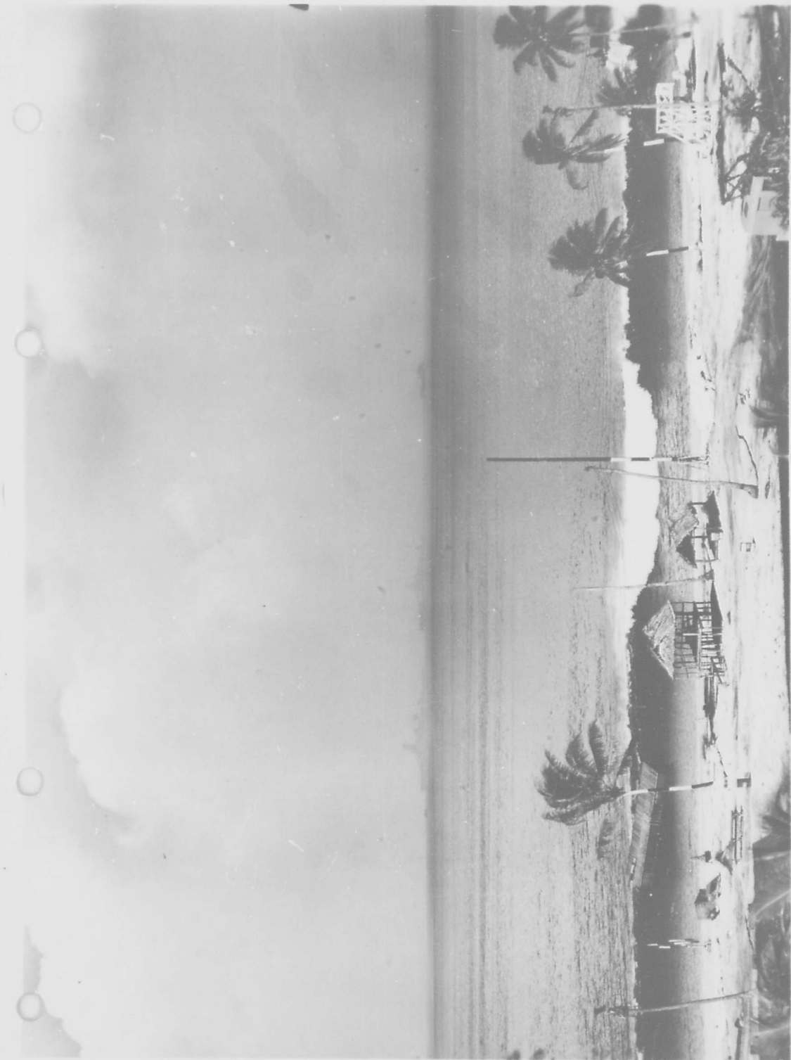
FIGURE 18 - FIRST WAVE COMMENCING TO BREAK OUTSIDE SWIMMING PONTOON. AT THIS POINT THE CREST WAS FIFTEEN FEET HIGH.
